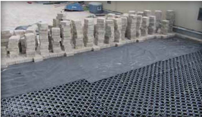
Figure 7. Concrete pavers on geotextile over plastic grids
