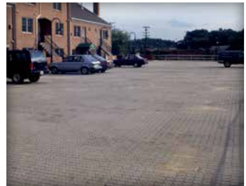
Figure 2. Concrete pavers serve vehicular traffic and parking over a concrete parking structure next to a residential development.
