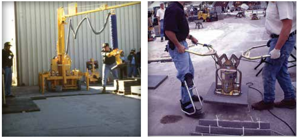
Figure 21. Vacuum assisted mechanical equipment for installing paving slabs.
