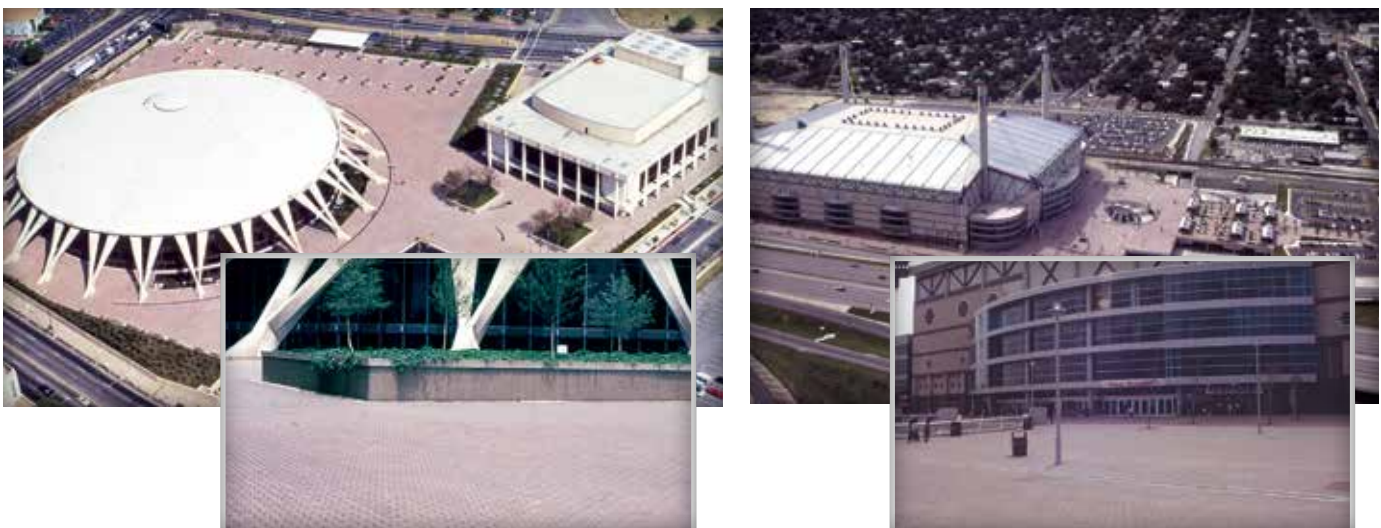
Figure 22. The plaza area around Scope Center in Norfolk, Virginia, (left) and one side of the Alamo Dome (right) in San Antonio, Texas, include roof plaza decks surfaced with concrete pavers.
