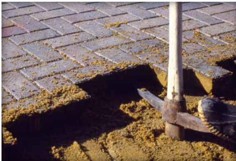
Figure 6. Prying out the remaining pavers
