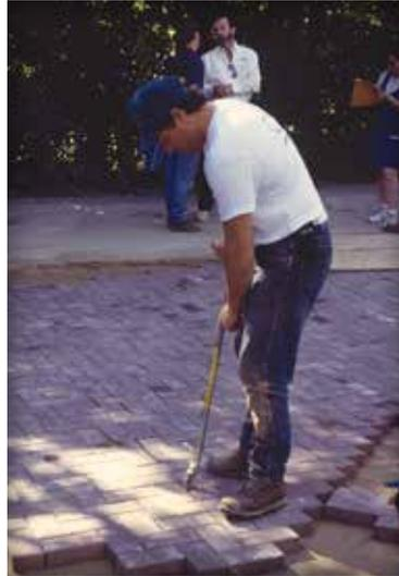
Figure 13. Adjusting joint spacing and alignment.
