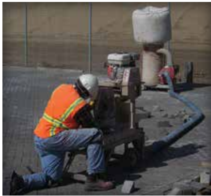
Figure 9. Edge pavers are saw cut to fit against a drainage inlet.
