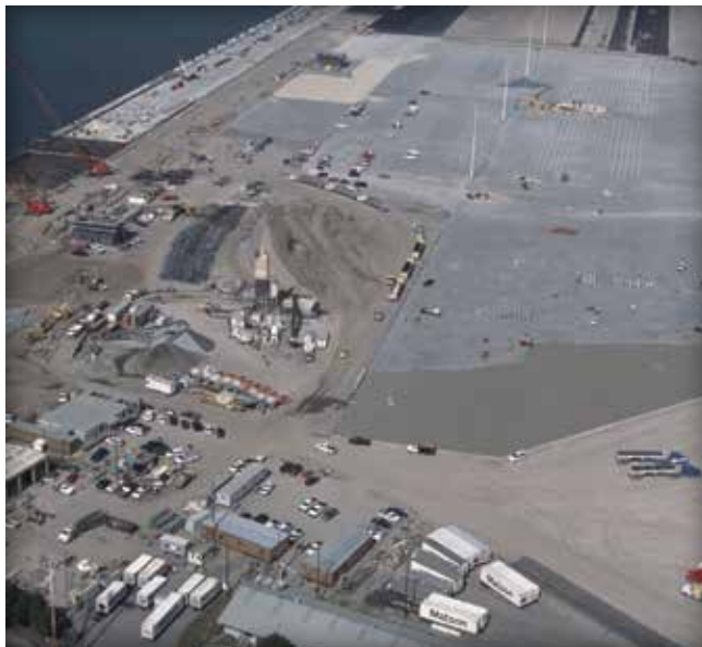
Figure 14. The Port of Oakland, California, is the largest mechanically installed project in the western hemisphere at 4.7 million sf (470,000 m 2 ).
