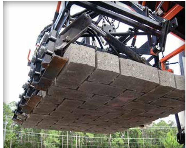
Figure 3. A cluster of pavers (or layer) is grabbed for placement by mechanical installation equipment. The pavers within the cluster are arranged in the final laying pattern as shown under the equipment.
