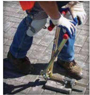
Figure 11. During initial compaction, cracked pavers are removed and immediately replaced with whole units.
