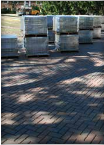
Figure 2. Bundles of ready-to-install pavers for setting by mechanical equipment. Bundles are often called cubes of pavers.
