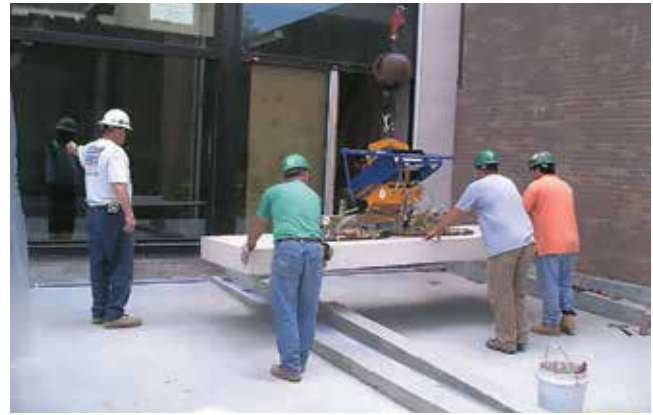
Figure 12. Large vacuum head lifts an oversize paving slab
