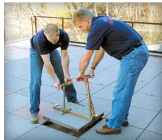
Figure 10. Double hand clamp for lifting larger paving slabs
