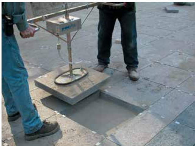
Figure 13. Two-person vacuum lift for paving slabs
