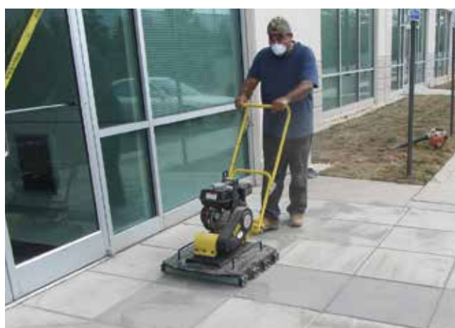
Figure 18. Compacting paving slabs with a roller attachment on a plate compactor
