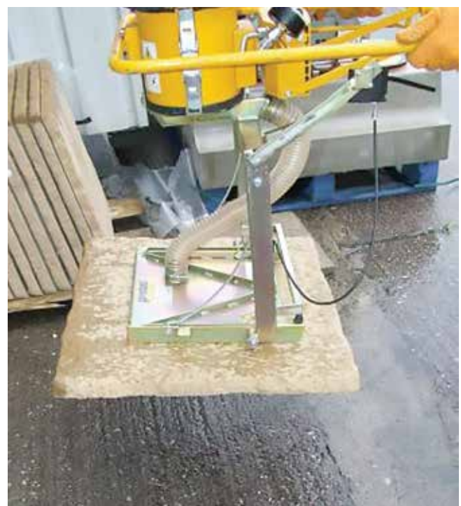
Figures 16 and 17. Vertically stacked paving slabs on a shipping pallet can be lifted, turned to a horizontal position and placed with a vacuum device.
