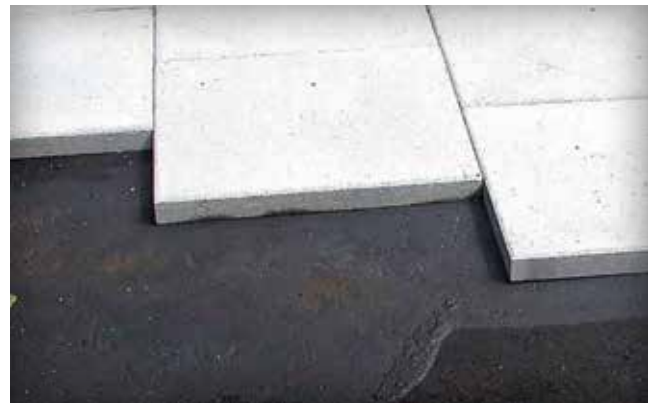
Figure 7. Sidewalk application illustrating the neoprene adhesive on an asphalt bedding layer under paving slabs
