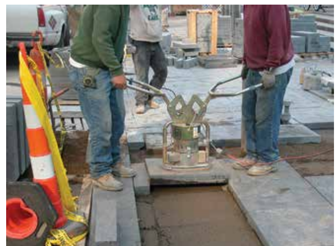
Figure 14. Two-person vacuum lift for larger paving slabs.
