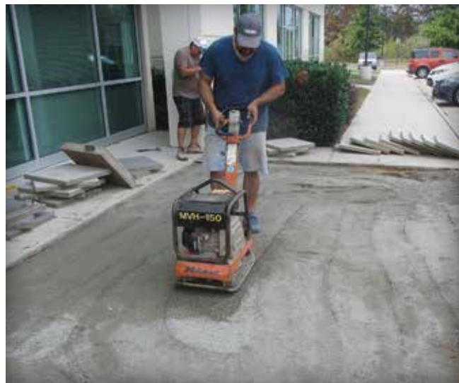
Figure 5. Precompacting the bedding sand
